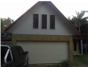
Above: A recent renovation project completed by B.A. Fisher Building
